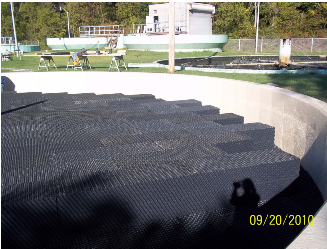
Figure 2. Cross Flow Installation
