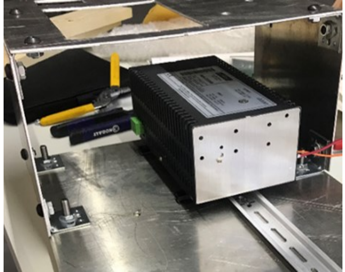
Figure 5. Installing DIN rail and LinMot power supply.
