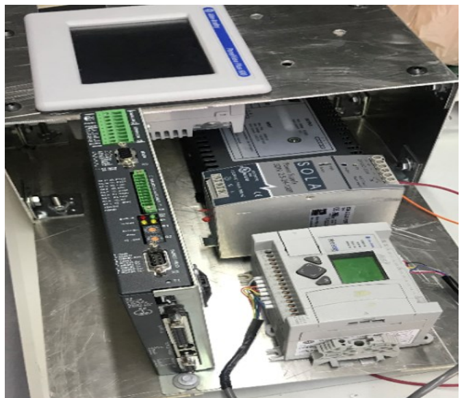
Figure 6. Installing all system components.
