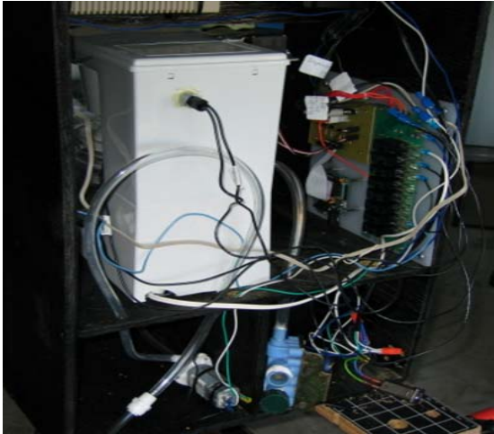
Figure 6. Vinyl tubing, drain pump, and solenoid valve
