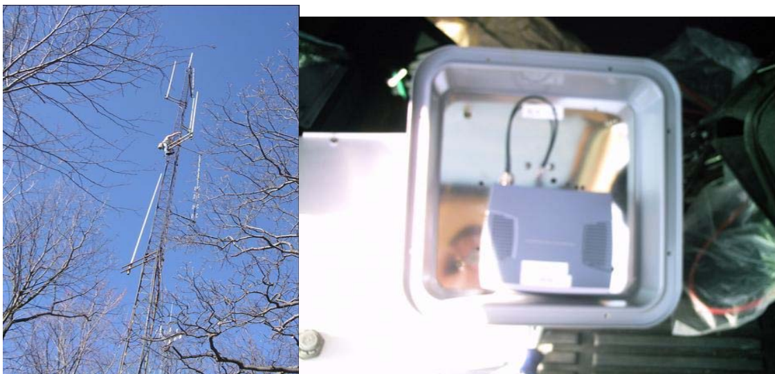
Figure 10: The Bridge and its installation on the tower
