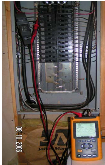
Figure 2 Power analyzer connections
