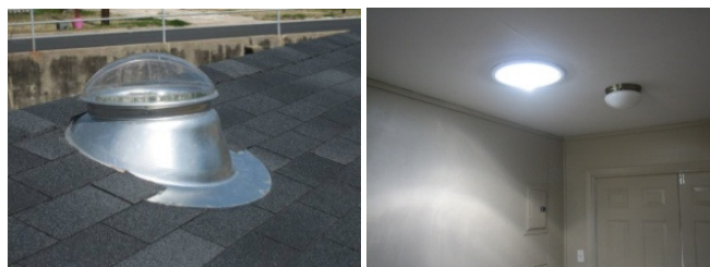
Figure 1. Skylight Installation
