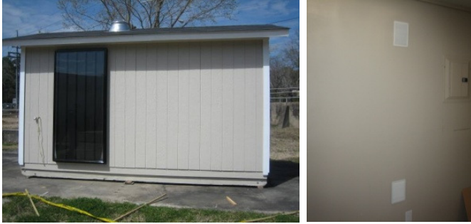
Figure 2. Passive Solar Air Heating System
